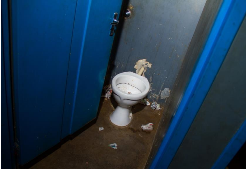
Fig 1. Restrooms at the Tutugeni Open Market in Okuryangava
