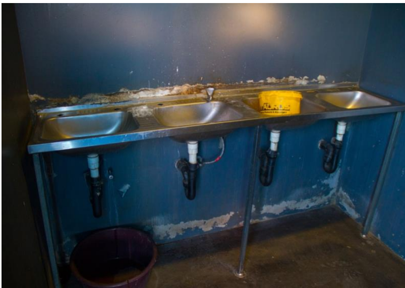
Fig 2. Restrooms at the Tutugeni Open Market in Okuryangava
