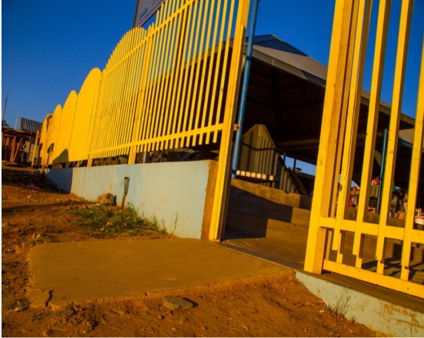
Fig 5. Accessibility ramps at the Lyeeta Market, Okuryangava
